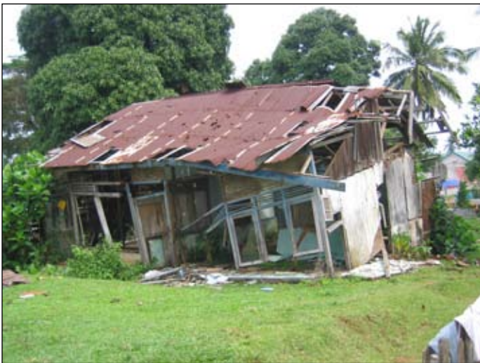
Figure 10. Timber frames with masonry skirt, Kec. Lais (North Bengkulu). Left: Superstructure has shifted off, although the relatively heavy roof structure remains largely intact, and the masonry panel is partially collapsed, Kota Agung, S3.55841° E102.08951°.
