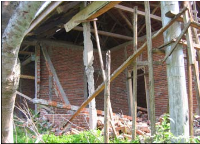
Figure 3. Confined masonry houses with failure in masonry walls and connections between tie columns and bond beams, Kec. Airnapal (North Bengkulu).
