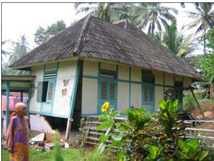
Figure 10. Timber frames with masonry skirt, Kec. Lais (North Bengkulu). Left: Superstructure has shifted off, although the relatively heavy roof structure remains largely intact, and the masonry panel is partially collapsed, Kota Agung, S3.55841° E102.08951°.
