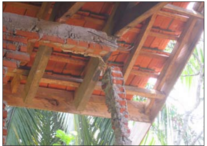
Figure 3. Confined masonry houses with failure in masonry walls and connections between tie columns and bond beams, Kec. Airnapal (North Bengkulu).
