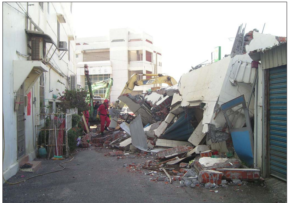
Figure 8. Side view of the collapsed furniture store.
