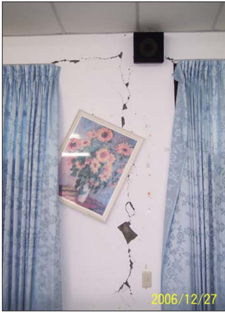
Figure 9. The damaged column along the corridor.
