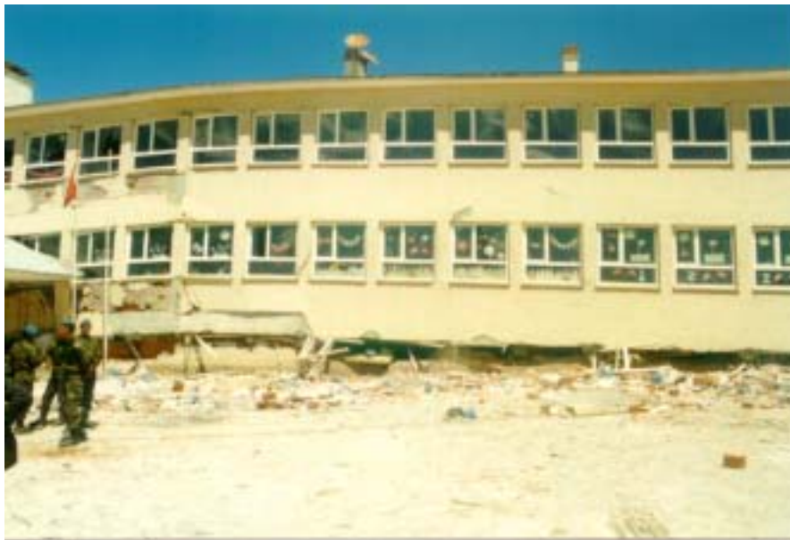
Figure 15. Çeltiksuyu Regional Primary Education School Building (Note identical entrance canopy partially visible on left. Again, the ground story had collapsed fully in exactly the same way as that in Figure 14. This building had been completed in 1998.)
