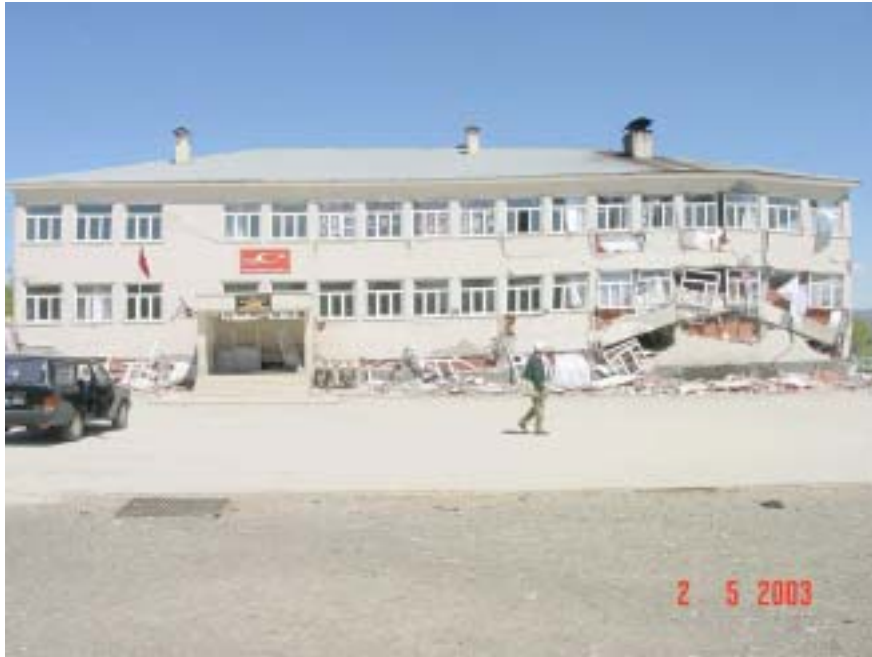
Figure 14. Kaleönü Primary Education School Building (This school is located 7 km to the west of the one in the next figure, but has an identical design. It is located at the city fringe. Note the canopied entrance that is now at the second story level. The story mechanism appeared to have been triggered by flexural action. Column reinforcement was plain bars, transverse confinement in columns negligible, and nonexistent within joints.)
