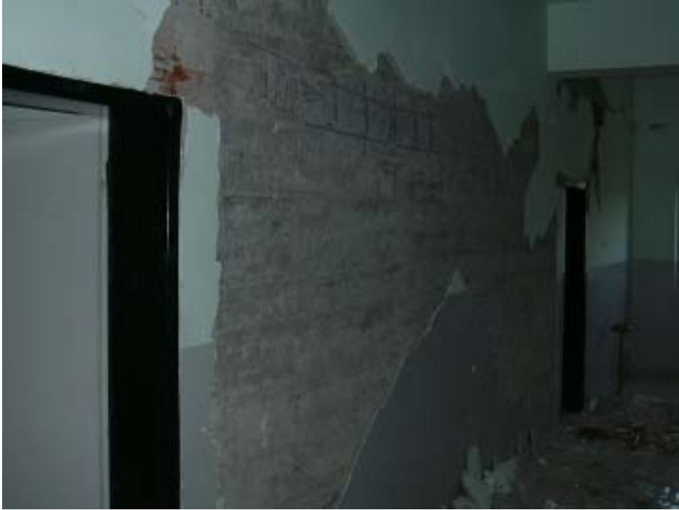
Figure 22. Just-Completed High School Building in City (The two shear walls flanking the hallway are the only ones in the longitudinal direction. Wall facing this one damaged worse. The only wall in the transverse direction appeared to be in a state similar to this. Source: Dr. E. Karaesmen.)
