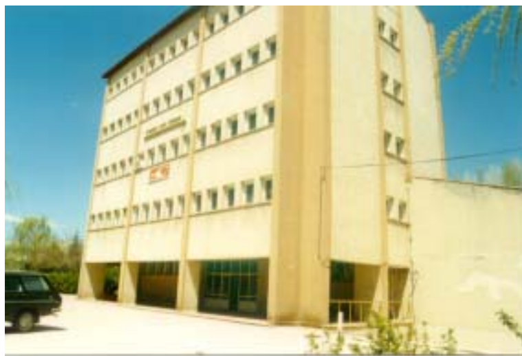
Figure 5. Ministry of Public Works and Settlement Regional Office in Bingöl (The recording instrument was in the back of the adjacent building.)
