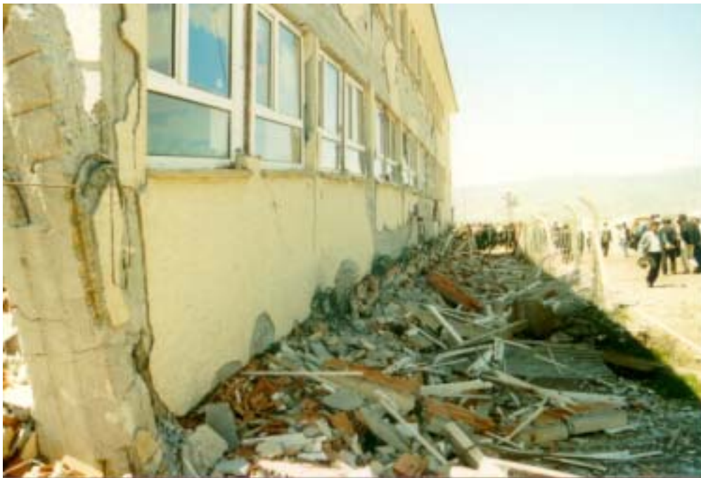
Figure 17. North Side of Building in Figure 15
