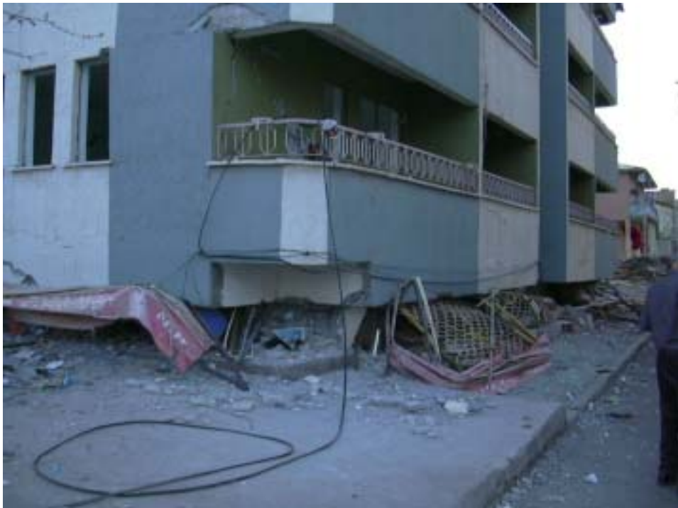
Figure 23. Another Recently Completed Building That Experienced Ground Story Failure (Source: Dr.E. Karaesmen)
