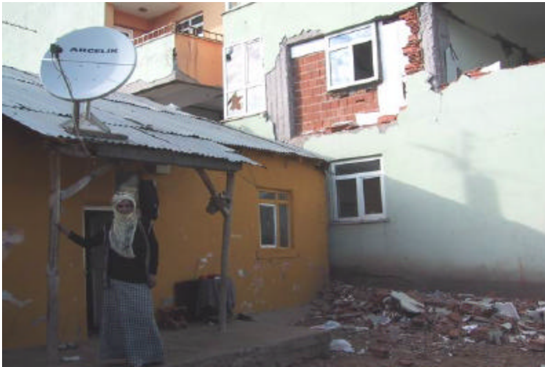
Figure 2. In Central Bingöl, life in a one story house adjacent to a heavily damaged high rise building (Photo: A. Nuray Karanci)
