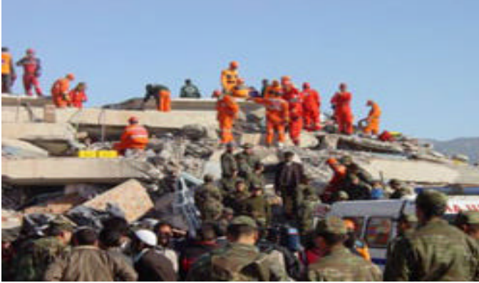
Figure 1. Çeltiksuyu Regional Boarding School Dormitory Building : Search and Rescue
