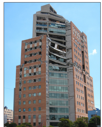
Partial collapses in an RC-wall building in Concepción, Chile, 2010 (photo: J. Mitrani-Reiser).
