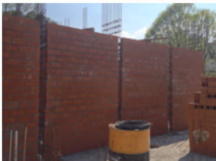
Figure 1. Masonry wall construction
