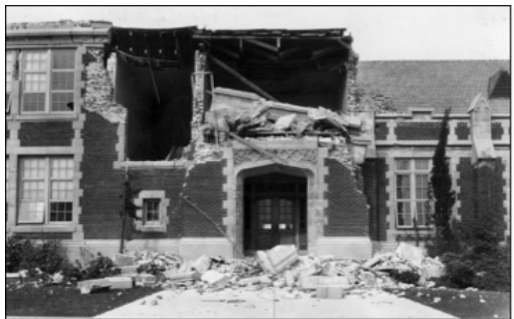
View of John Muir School, showing damage from the March 10, 1933 Long Beach earthquake. Located on Pacific Ave. in Long Beach, California. Photo taken 8 days after, on March 18, 1933. (photo: W.L. Huber, source: USGS, 1993).
