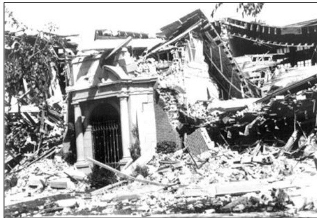
Fig. 6 – Jefferson Jr. High School in Long Beach, California, destroyed by the March 11, 1933 earthquake [15].
