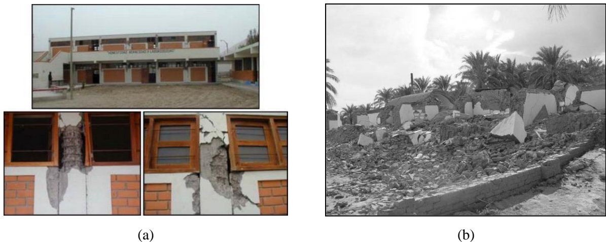
Fig. 1 Vulnerability and deficiencies problems presented in school buildings during earthquakes: (a) Captive columns in schools in Perú (Figure 18 from reference [4]); (b) Adobe school totally collapsed in Iran (Figure 6a from reference [6]).
