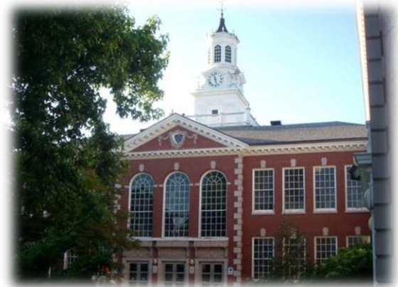
A typical unreinforced masonry high school in the United States. (Wang, Y., EERI, 2012a)
