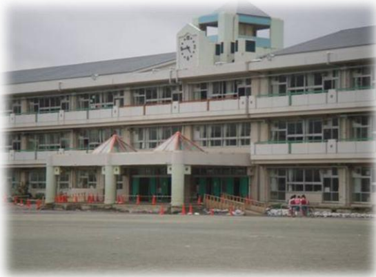
This Japanese school is in session after the 2011 Tohoku earthquake. Notice the evidence of liquefaction and settlement around the building. The building used pile foundations and was built for seismic conditions. (Wang, Y., EERI, 2012b)
